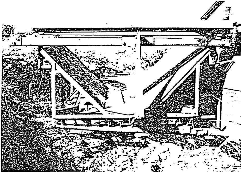
Fig. 1a. Typical slot sampler as installed on a  $1.4 \text{ m}^3 \text{ s}^{-1}$  super critical flume. The downstream view shows the moveable and fixed slots, the flume, and the bottle storage mechanism house.
