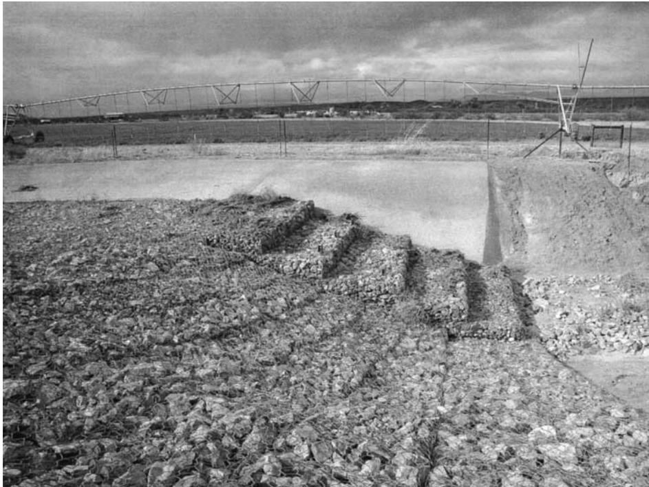
**Fig. 1** Stair stepped gabions, wire mesh, and concrete reinforced bank controlling erosion on the edge of an irrigated field in southern Arizona.
