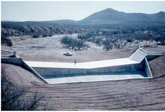
Figure 2. The hydraulic measuring device and energy dissipater at the outlet of Walnut Gulch [Gwinn, 1964; Smith et al., 1982]. The photograph was taken prior to any flow through the measuring station.
