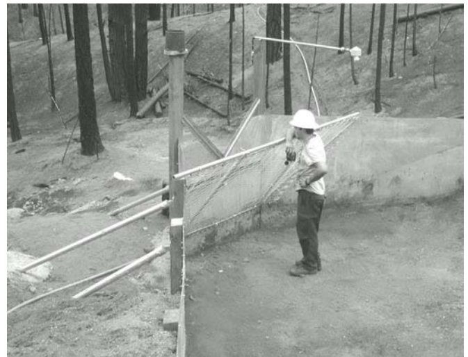
Figure 3. V-notch weir and trash/debris screen.
