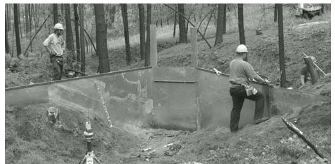
Figure 2. Sidewalls of sediment trap.
