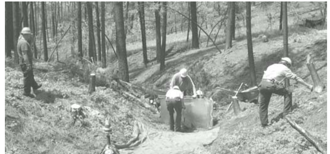
Figure 1. Sheet metal cut-off wall installation.
