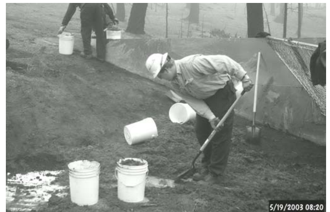
Figure 4. Buckets are used for sediment clean out.
