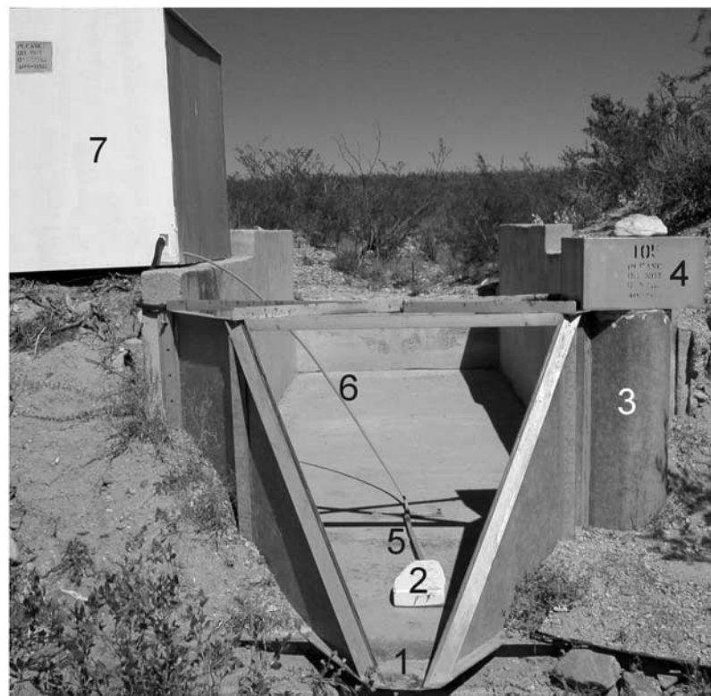
Figure 1. View of H flume at LH105 showing (1) flume exit, (2) float that raises perforated sediment sampling tube in response to water level, (3) stilling well, (4) water level instrument house, (5) sediment intake tube, (6) pump sampler tube, and (7) housing for pump sampler.
