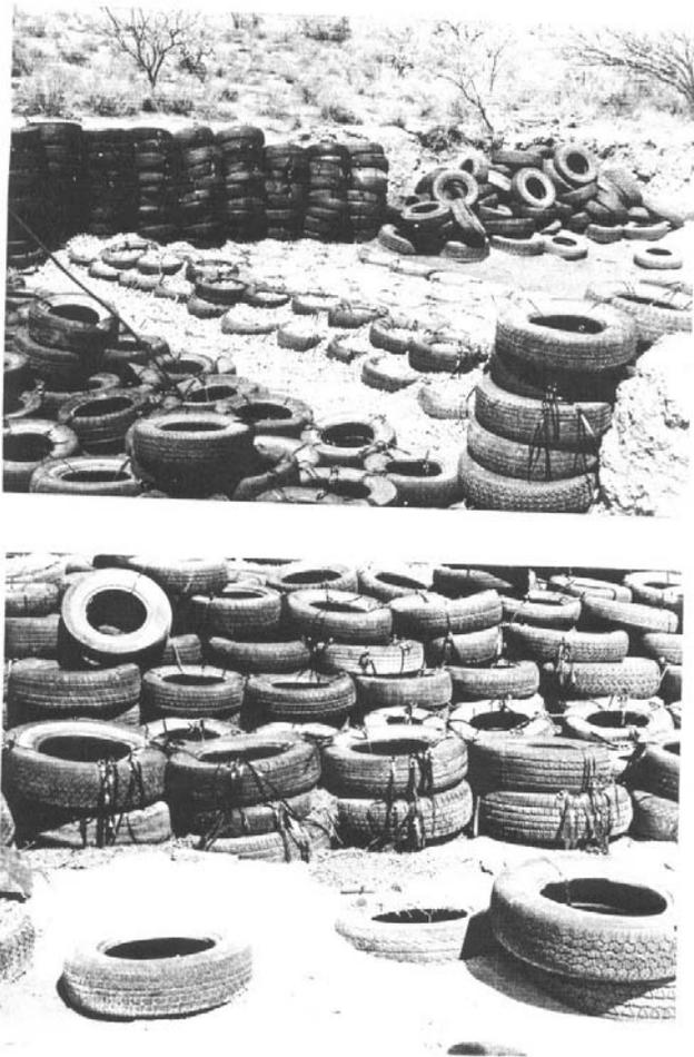
Figure 1. Erosion control dam under construction.
